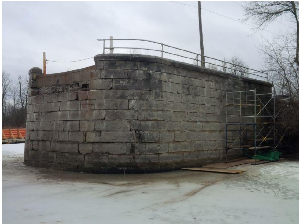
The historic masonry making up the bridge abutment will also be repaired
