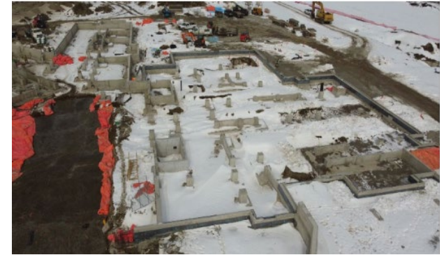
Overview of Work Progress
