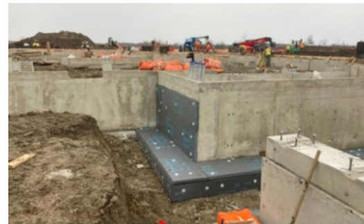
Insulation work around footings
