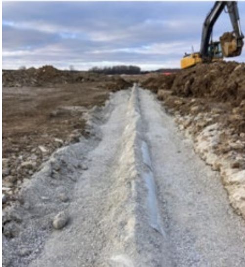
Septic Field Drainage & Storm water piping
