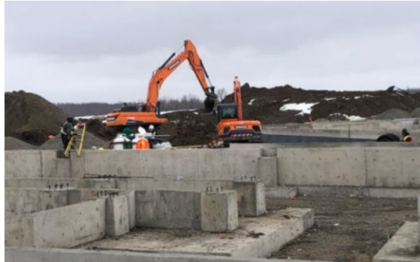
Foundation Works stripped in North / West wing
